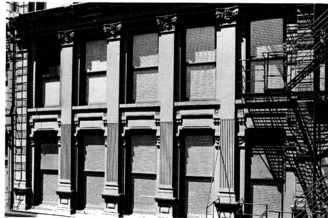
The two-story-tall "pilasters" on the Haskell and Barker Buildings are rare examples of classical-style detailing on an 1870s Loop commercial building.
